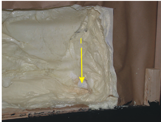
I. Electrical Conduit After Trimming
